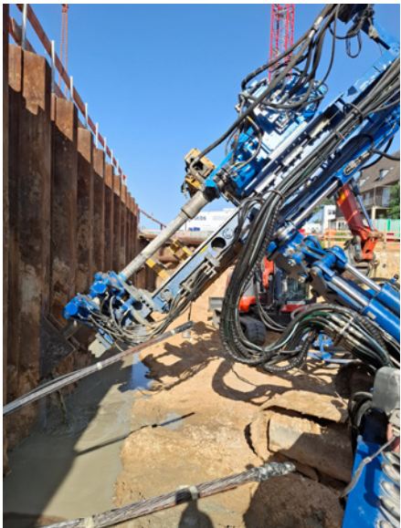
VD 100 drilling hole diameter 114 mm, 13,5 m deep for strand anchors near a hospital.
