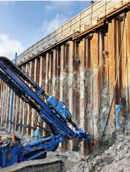
VD 150: production of stranded anchors, 30 m long.
