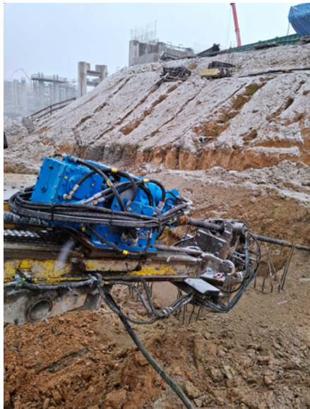
VD 50 drilling hole diameter 76 mm, 20 m deep for strand anchors.
