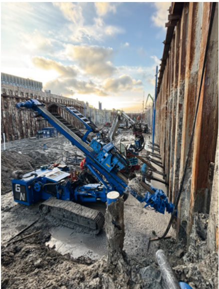
Drilling 73 mm selfdrilling hollow bars 65 m deep into sand and gravel.
