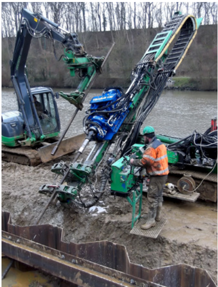
VD 150 drilling hole diameter 152 mm, duplex with inner rod 30m deep for strand anchors in different soil layers from clay to lime and flintstone.
