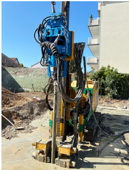
VD 50 drilling hole diameter 200 mm near for concrete posts.
