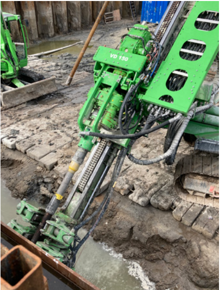
VD150 drilling 177.8 mm casings for strand anchors, 60 m long.
