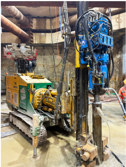
VD 50 drilling hole diameter 201 mm for pilot holes in the concrete and gravel soil.
