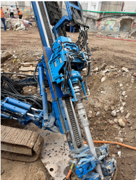
VD 100 drilling hole diameter 133 mm duplex casing and inner rod, 20 m deep for strand anchors in clay soil.
