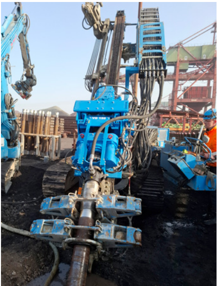
VD 150 drilling hole diameter 177,5 mm, 25 m deep in sand / gravel soil.
